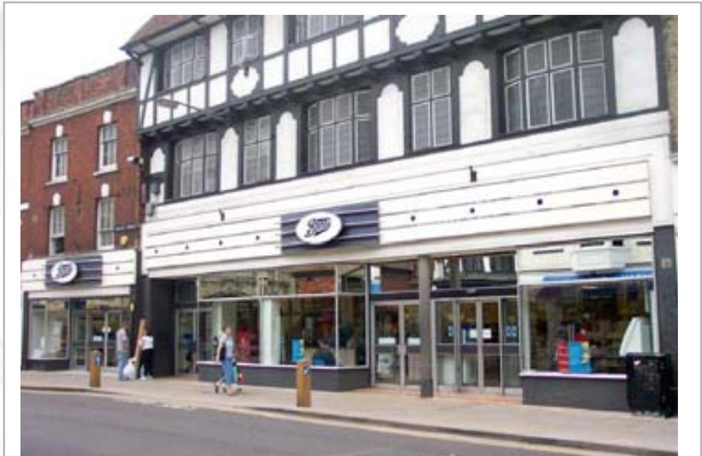
**Fig 11:** A shopfront with a wide expanse of flat glass. The fascia is made of modern materials and is overly large, impinging on the first floor. The shopfront does not reflect the architecture and the rhythm of the upper floors and the fascia is overbearing.
